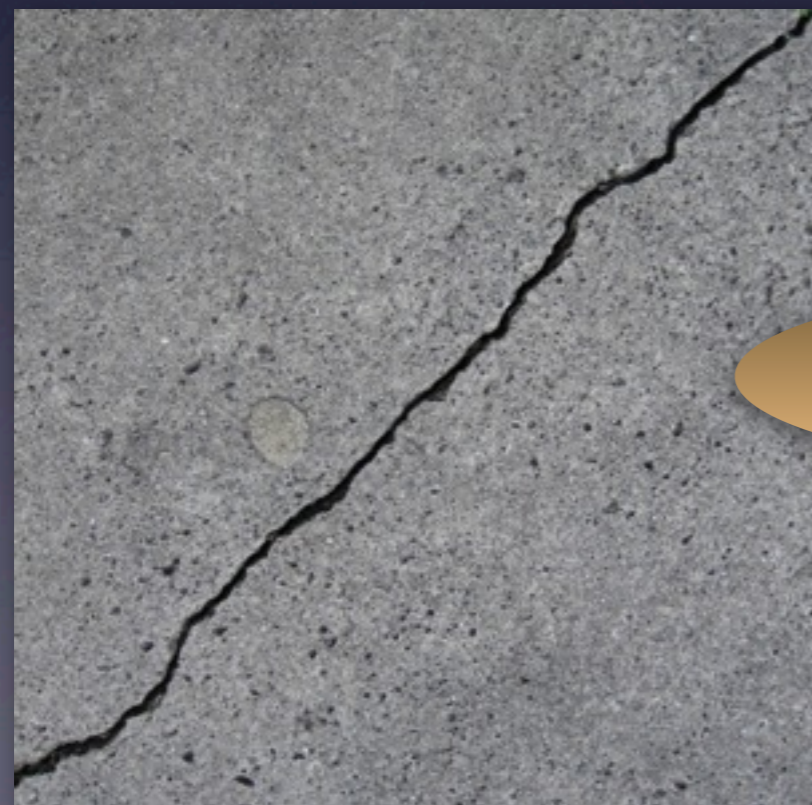
← Crack in a pavement
